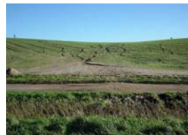
Examples of rill erosion and re-deposition of sediment at the base of the slope
