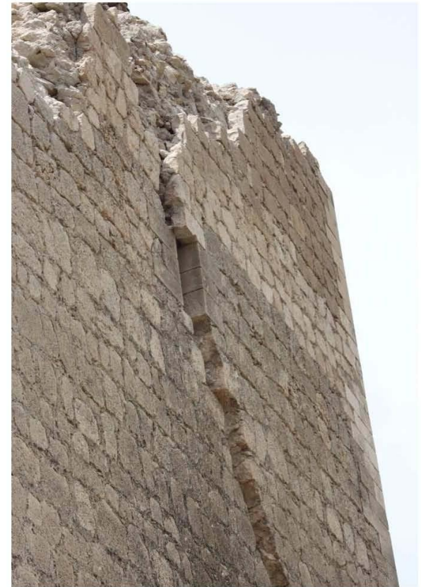
Shear crack onto the castle tower – sliding toward north direction
