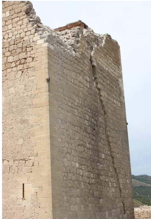
Shear crack onto the castle tower – sliding toward north direction
