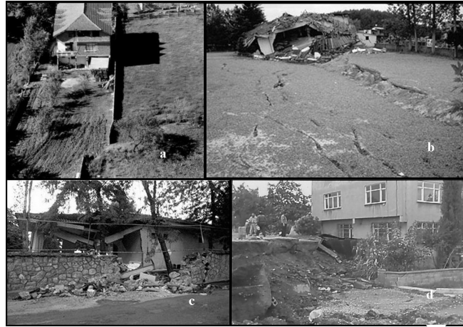
Fig. 4.1. Effects of fault rupture on buildings
