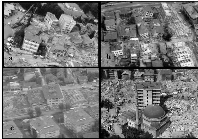
Fig. 4.2. Variation of building damage in different zones in the near field during 1999 Kocaeli, Turkey earthquake
