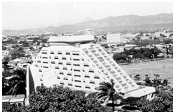
Fig. 13.1. This building successfully withstood the great Managua earthquake, thanks to its suitable distribution of masses, although someone had the idea of placing a large water tank on the roof, supported on a floor of columns that collapsed, and after the earthquake it was observed that the water tank had come to rest directly on top of the lower structure
